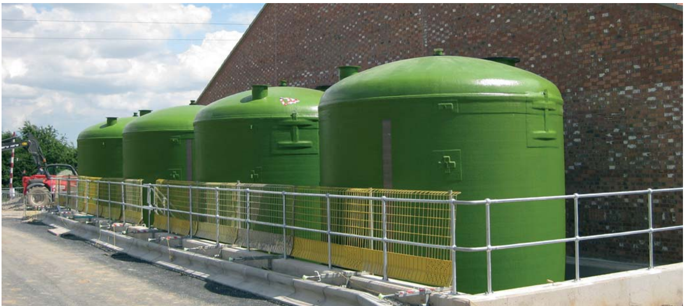
New Building with Saturators being Installed
