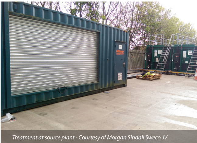
Treatment at source plant area - Courtesy of Morgan Sindall Sweco JV
